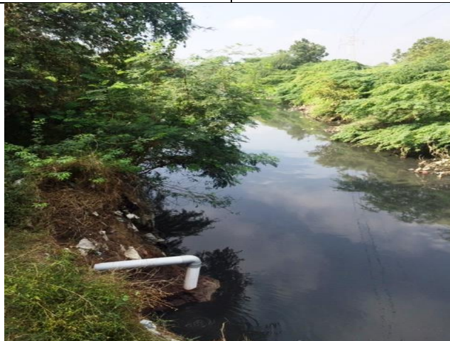
Discharge line at the backside of Surajmani corporation in Khari River
