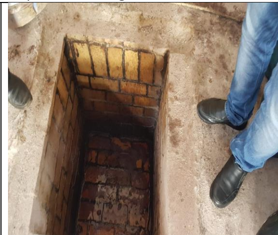
Discharge Pit in the production area
